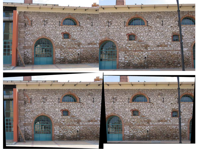
Figure 9. Final rotated images of the above pair (image axes convergence of 10^\circ ).
