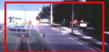
Example of a frontage lane built in the 1960's. Stop signs have been added to frontage road due to confusion on right of way.
